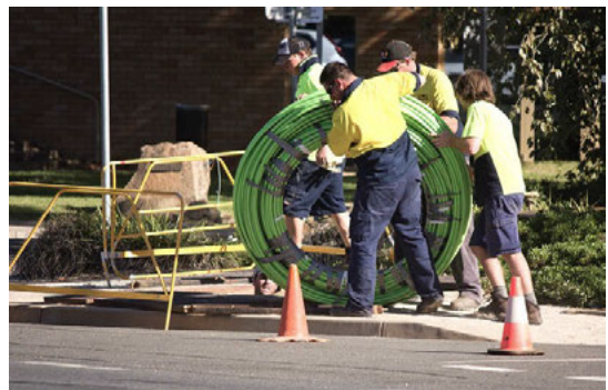
NBN fibre-optic cable being laid; photo: Bidgee
