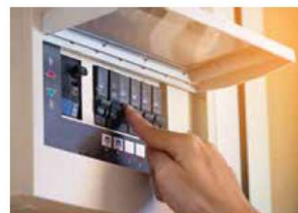
Figure 2 Resetting a circuit breaker switch in the distribution board. The switch in the up position means it is closed, so the circuit can operate.
