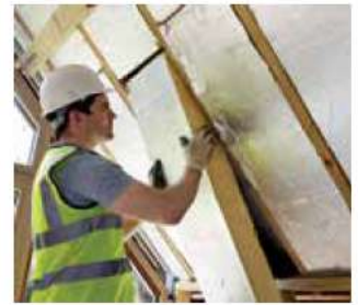
Figure 8 A builder installing insulation in a roof. The material is a poor conductor and it has a reflective surface to reduce radiation.
