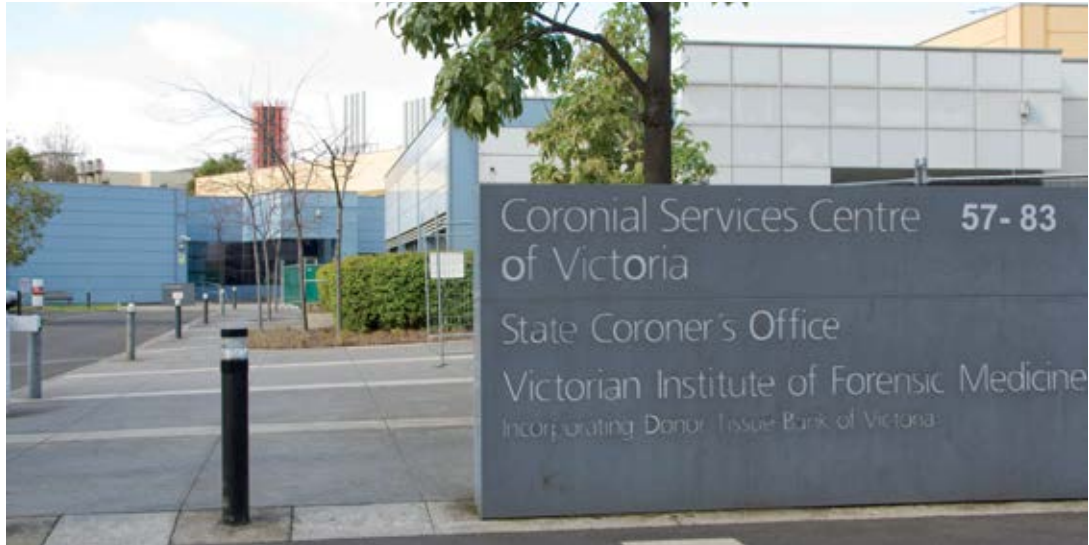
Figure 4.8 The Coronial Services Centre
